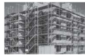
Fig. 5: Structural shell Masonry building, under construction
