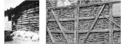
Lattice + clay Beam- and framework construction
