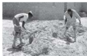
Fig. 2: Earth Mixing with cob and sand
