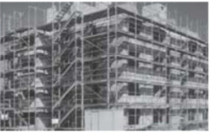
Fig. 5: Structural shell Masonry building, under construction
