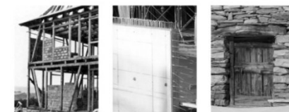
Beam- and framework construction Infill with masonry
