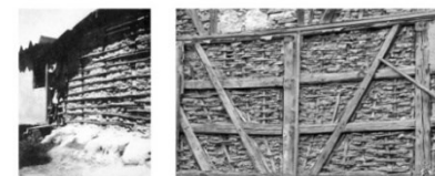
Lattice + clay Lattice construction with clay
