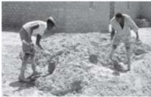
Fig. 2: Earth Mixing with cob and sand
