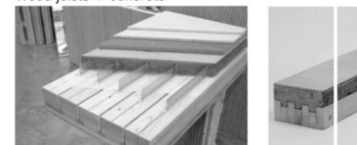
Wood - concrete composite slab Composition through metal slices
